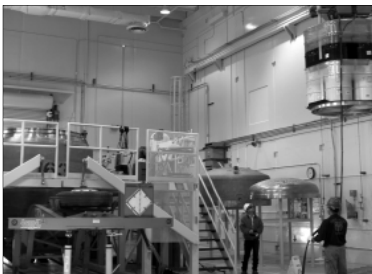
WIPP waste handling building.
