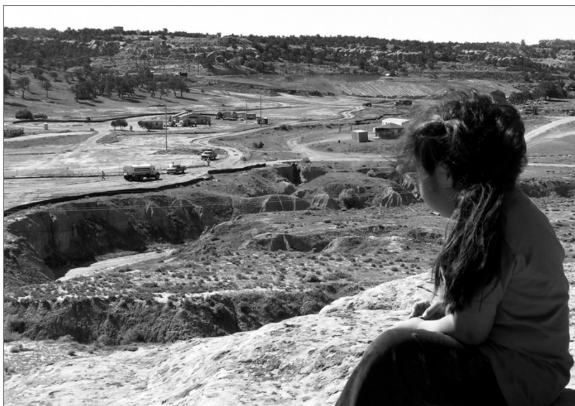
A grandson of Teddy Nez watches the equipment remove soil as part of the 2009 "removal action."
