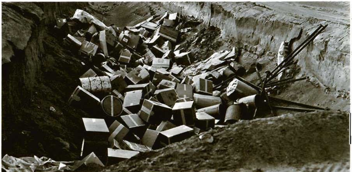
Radioactive waste was buried in shallow trenches at Hanford through the mid 1980's.
