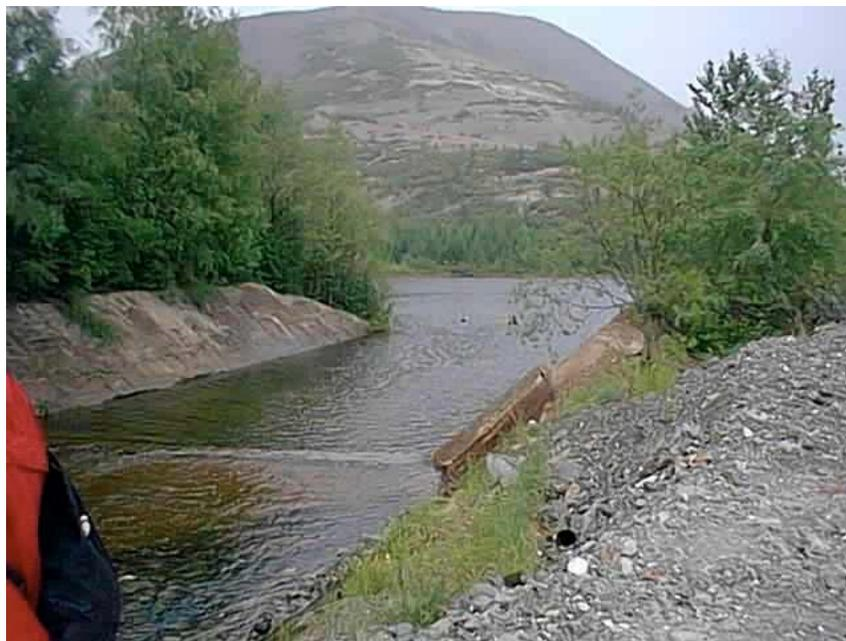
**View of Inlet to Diversion Channel without Pillars to Prevent Intrusion of Ice into Diversion System**
