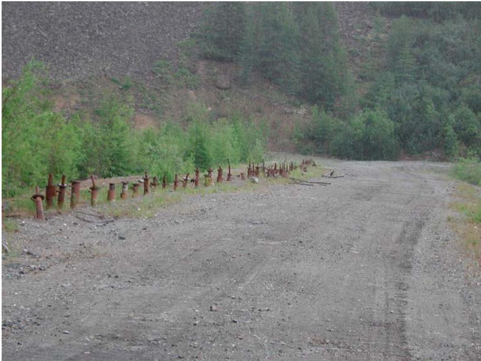
**View of Vandalized Thermistors Designed to Keep Upstream “Head” Dam at Karamken Frozen**
