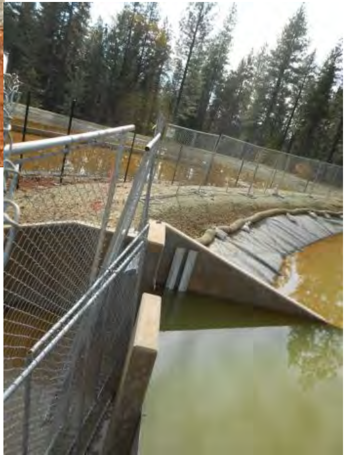
2 - Outfall from Settling Pond to Wetland No.1
