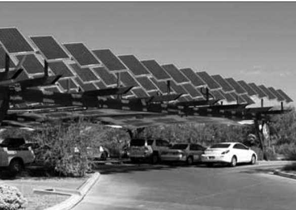
the visitor parking lot at Springs Preserve in Las Vegas, Nevada.
