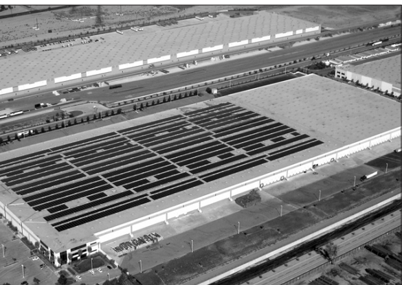
Edison installed "thin film" solar photovoltaic panels on a rooftop of a Fontana warehouse. Photo courtesy of Edison.
