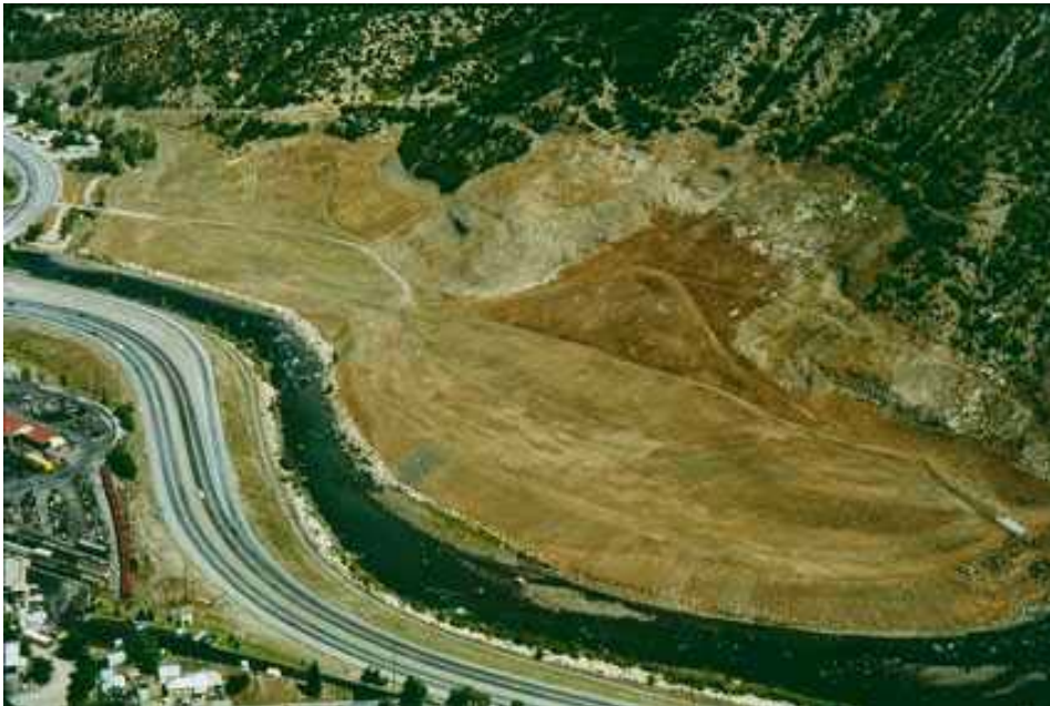
PHOTO 2 – Durango, CO UMTRAP Site after removal of all tailings, residual contamination and covering with radon barrier, 1991.
