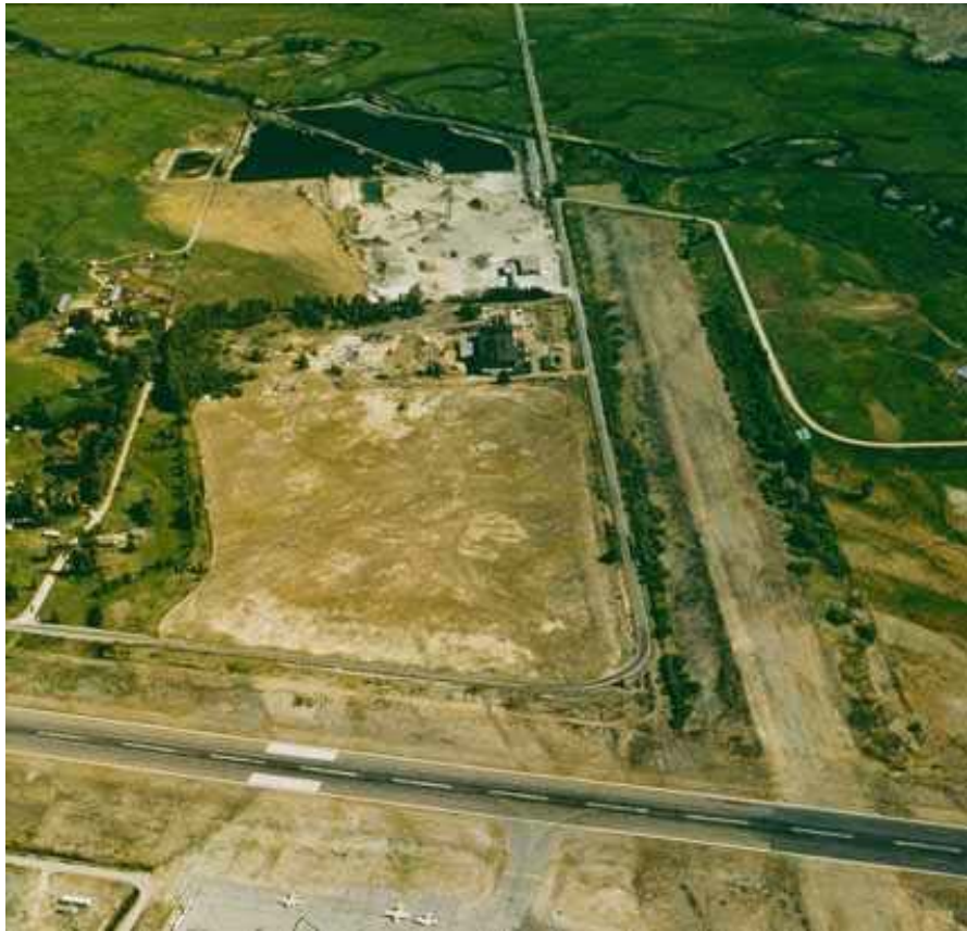
PHOTO 8 – Gunnison, CO UMTRAP site following surface remediation in place, 1995
