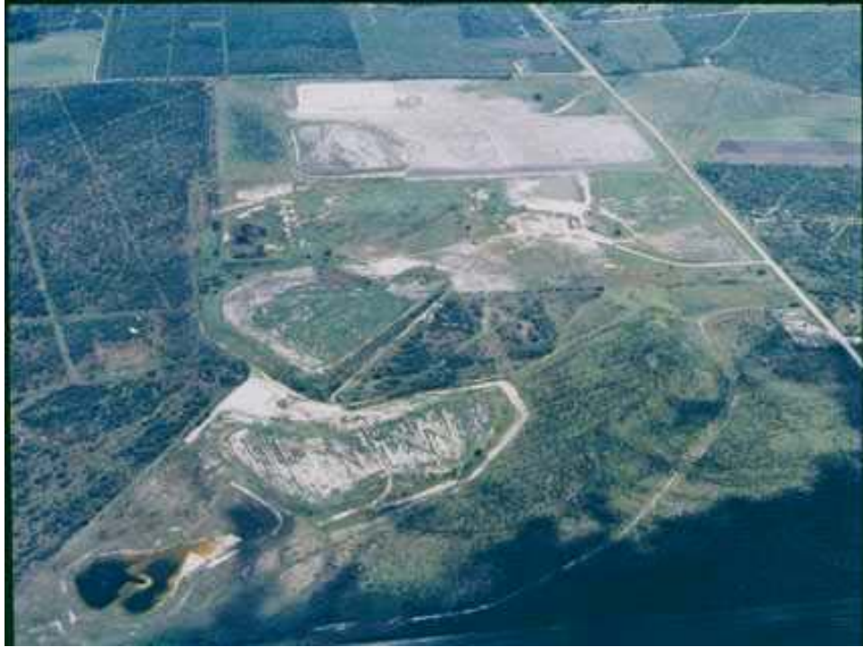
PHOTO 5 – Falls City, TX UMTRAP Site prior to remediation, 1987
