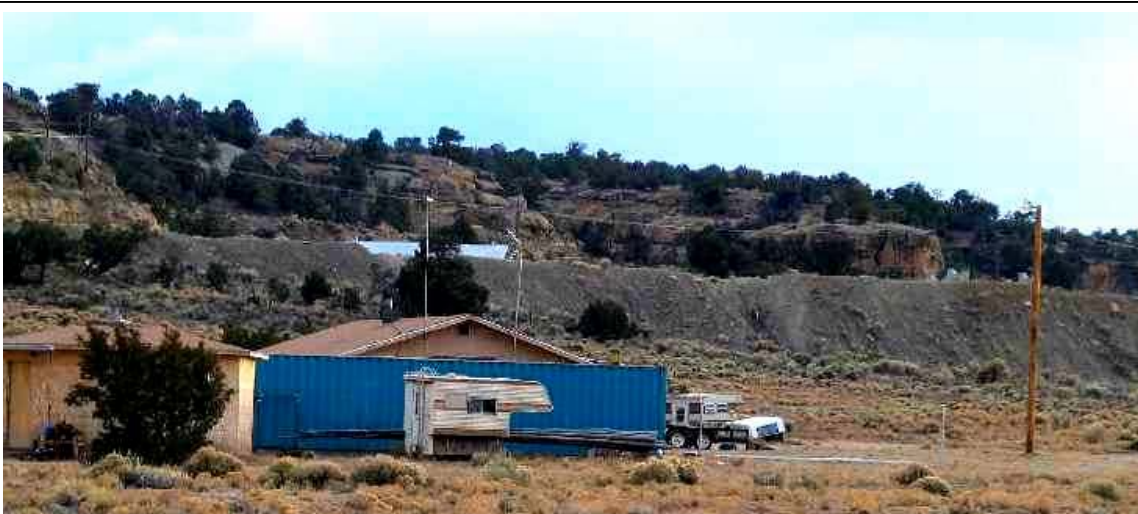
Figure 3. Navajo residence within 600 feet of NECR Mine waste dump, 2005.
