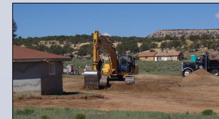
Backhoe removes soil around hogan, May 2007
