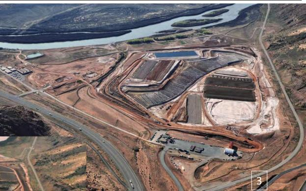
From: <u>http://www.gjem.energy.gov/moab/</u> and <u>http://www.moabtailings.org/</u> Crescent Junction Disposal Site uses below-grade tailings disposal with windborne particles releases controlled daily cover using material excavated to allow below grade disposal.
