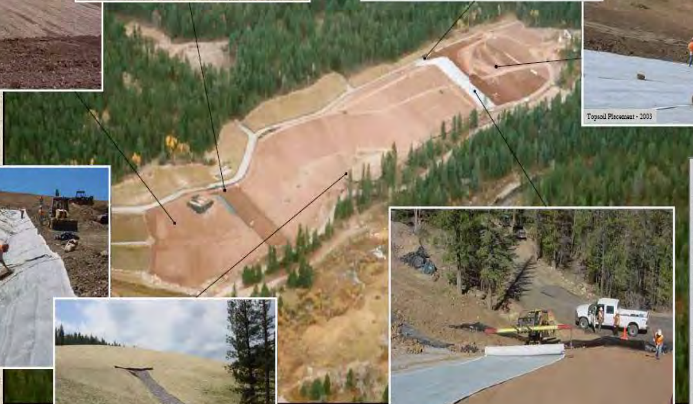
Anchor Trench Construction - 2003
