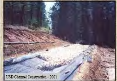
USD Channel Construction - 2001
