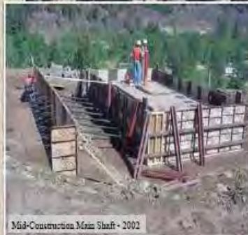
Mid-Construction Main Shaft - 2002
