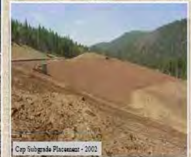
Cap Subgrade Placement - 2002
