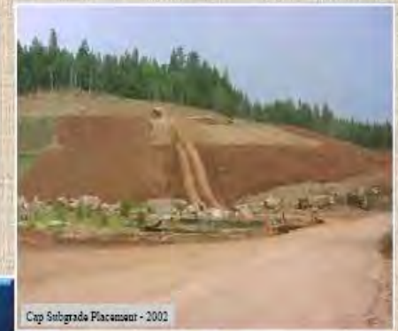
Cap Subgrade Placement - 2002
