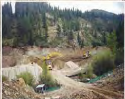
Willow Creek Waste Rock Excavation - 1999
