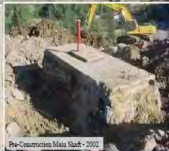
Pre-Construction Main Shaft - 2002
