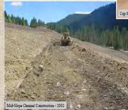
Mid-Slope Channel Construction - 2002
