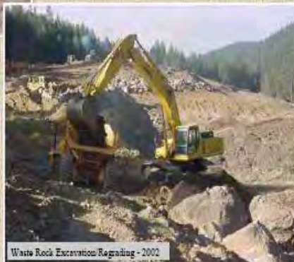
Waste Rock Excavation Regrading - 2002
