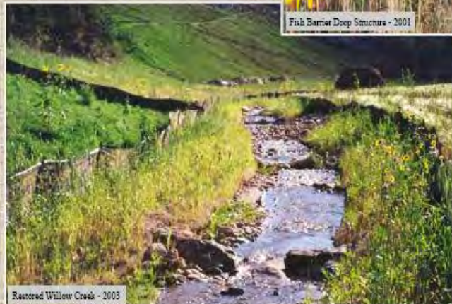
Restored Willow Creek - 2003
