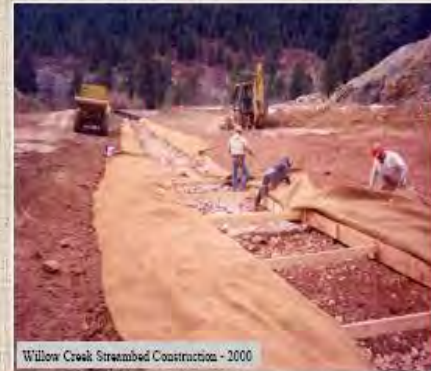
Willow Creek Streambed Construction - 2000
