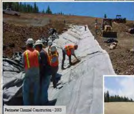
Perimeter Channel Construction - 2003
