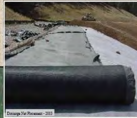
Drainage Net Placement - 2003
