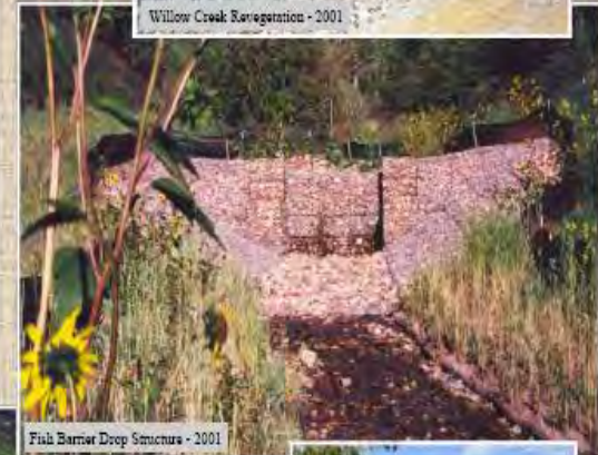
Fish Barrier Drop Structure - 2001
