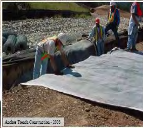
Anchor Trench Construction - 2003
