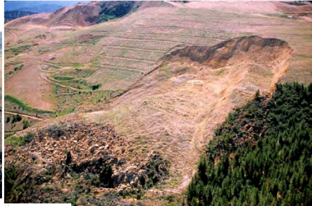
Photo 2. Aerial view of 1996 slide area. Note native bedrock material at toe of slide.
