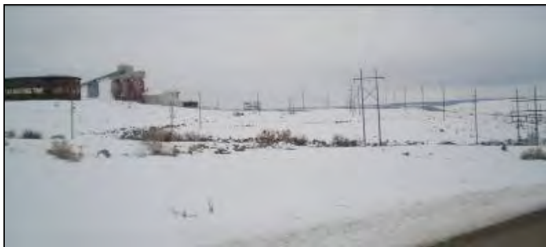
Power lines and other infrastructure in place at the Black Mesa Coal Mine
